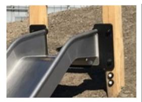
Slide interface panel of 19mm EcoCore™ which a highly durable, eco-friendly material, which is not only recyclable after use, but also consists of a core produced from 100% recycled material.
