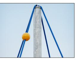
In the center of the net is the mast, made of high quality seamless steel. The structure of the mast as an oscillating support is statically favorable and equalizes the oscillations in the net. The masts are hot dip galvanized as standard, with the design option of additional powder coating.
