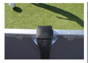
The posts are made of 80 x 80 x 3mm profile with horizontally, 6mm welded flanges. This will enable an easy installation and strong construction. The low-density polyethylene post caps are attached with blind rivets.
