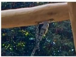
Swing hangers for Robinia wood crossbeams are made of stainless steel brackets and can move over two axes. The flange bearings are silicone enriched to make the suspension maintenance free.
