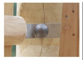
The hardware is made of stainless steel or galvanised steel to ensure durable connections that has high corrosion resistance.
