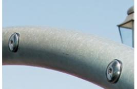
The steel structures are hot-dip galvanised inside and outside with lead free zinc. The galvanisation has excellent corrosion resistance and requires low maintenance.
