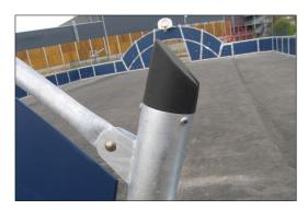
Pole tops are molded of thermoplastic rubber (TPV) with a steel inlay. TPV is highly durable against wear and tear, and the steel inlay secures durability.
