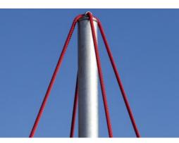
In the centre of the net is the mast, made of high quality seamless steel. The structure of the mast as an oscillating support is statically favourable and equalizes the oscillations in the net. The masts are hot dip galvanised as standard, with the design option of additional powder coating.
