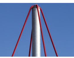
In the center of the net is the mast, made of high quality seamless steel. The structure of the mast as an oscillating support is statically favorable and equalizes the oscillations in the net. The masts are hot dip galvanized as standard, with the design option of additional powder coating.
