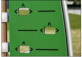
Panels of 19mm FcoCore™. FcoCore™ is a highly durable, eco friendly material, which is not only recyclable after use, but also consists of material produced from +95% recycled post consumer material from food packing waste.
