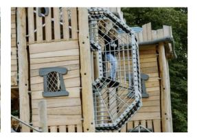
The wire frame tunnel is made of hot dip galvanised high quality steel. Corocord 16mm ropes are special 'Hercules'-type with galvanised four-stranded steel wires and a steel wire core. Each strand is tightly wrapped with PES yarn, which is melted onto each individual strand.
