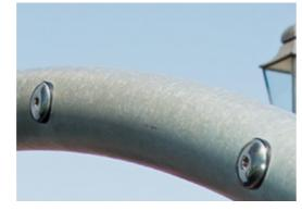
The steel structure are hot dip galvanised inside and outside with lead free zinc. The galvanisation has excellent corrosion resistance in outside environments and requires low maintenance.
