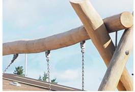
The swing hangers are made of high quality UVstabalised nylon (PA6) housing with integrated lifetime sealed ball bearings. The height adjustable chains are fixed by a stainless steel hook with theft proof snake-eye bolt in a turn able anti twist housing.
