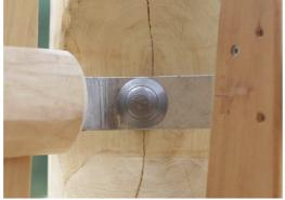
The hardware is made of stainless steel or galvanized steel to ensure durable connections with a high corrosion resistance.
