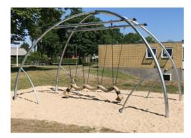
The steel pipes are hot-dip galvanised inside and outside with lead-free zinc. The galvanisation has excellent corrosion resistance in outside environments and requires low maintenance.
