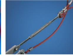
The spacenets' main bearing ropes are equipped with an additional safety feature: should the main connections fail, the safety rope prevents collapse of the structure.
