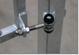
The hinges on the entrance gate are 16mm and made of Stainless Steel. The handles can be accessed from either side of the pitch.
