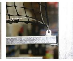
The net is made of a Ø4mm black polypropylene, better known as Nylon, with a mesh size of  $45 \times 45$ mm and reaches till 5m high. The nets will keep all balls in the MUGA and retains the transparency.
