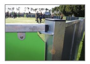
The HDPE panels are connected with M8 stainless steel bolts to  $42.5 \times 40 \times 3$ mm welded flanges. These connections are not visible from the inside and create a strong and safe connection.
