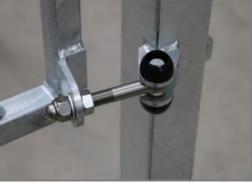
The hinges on the entrance gate are 16mm and made of Stainless Steel. The handles can be accessed from either side of the pitch.
