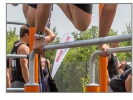
Bars intended as grips during exercises are made of hot-dip galvanised steel ø38mm. A great diameter to support the wrist when doing dips or handstands.
