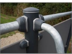
The connectors are made of die-cast aluminium.
