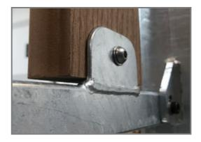
The WPC boards are attached to  $70 \times 45 \times 3$ mm welded flanges with stainless steel M8 bolts, nuts and washers. These connections are not visible from the inside and create a safe and robust connection.
