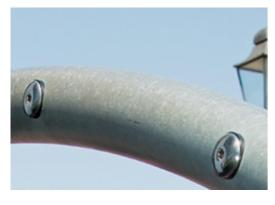
The steel structure are hot dip galvanized inside and outside with lead free zinc. The galvanization has excellent corrosion resistance in outside environments and requires low maintenance.
