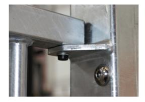
All steel components are manufactured from carbon steel, welding's according EN ISO 5817 & Hot dip galvanised (HDG) according to ISO1461. This process ensures good protection in all circumstances.
