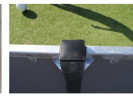
The posts are made of 80 x 80 x 3mm profile with horizontally, 6mm welded flanges. This will enable an easy installation and strong construction. The low-density polyethylene post caps are attached with blind rivets.
