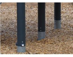
Main posts with hot-dip galvanised steel footing are available in different materials including; pressure impregnated pinewood posts, pregalvanised posts that are powder-coated or a lead-free aluminium option with an anodised colour top finish.
