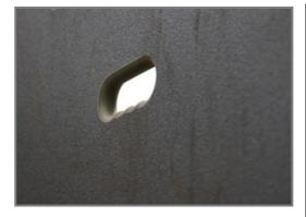
The wall surface are made of 17.8mm thick High Pressure Laminate (HPL) panels to ensure optimal strength and durability.
