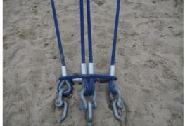
Huge spacenet structures are secured to the foundation with a system of three turnbuckles. Horizontal and vertical edge cables are fixed to individual turnbuckels, wich then connect to individual steel anchors. This system ensures that each edge cable can be tensioned separately and increases strucutral safety by way of independent anchoring.
