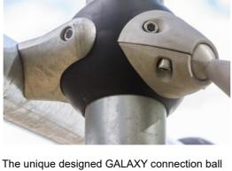
is made with an inner circular core of aluminium surrounded by a shell of hard PP with a outer layer of soft TPV rubber. Flexible lead free aluminium connectors allow for installation in variable angles.
