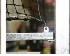
The net is made of a Ø4mm black polypropylene, better known as Nylon, with a mesh size of 45 x 45mm and reaches till 5m high. The nets will keep all balls in the MUGA and retains the transparency.
