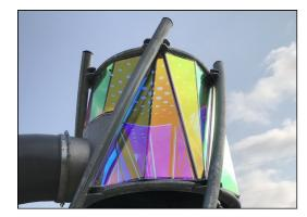
The graphic panels are made of high-quality polycarbonate with a thickness of 6mm. The colour changing dichroic film is glued on the outside. The PC panels are UV stabilized to prevent degradation.
