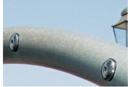
The steel arches are hot dip galvanized inside and outside with lead free zinc. The galvanization has excellent corrosion resistance in outside environments and requires low maintenance.
