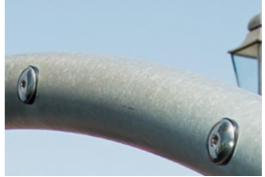
The steel structure are hot dip galvanized inside and outside with lead free zinc. The galvanization has excellent corrosion resistance in outside environments and requires low maintenance.
