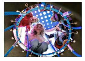
Corocord ropes of UV-stabilized PES rope strands with inner steel cable reinforcement. The polyester yarn is made from +95% post-consumer materials and is inductively melted onto each strand. PES has high strength with excellent resistance to abrasion and UV radiation. The ropes are connected by stainless steel S-Clamps which are pressed around the rope which results in a durable and vandalism solution.
