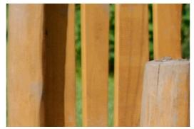
The Robinia wood can be supplied as untreated raw wood or painted with a brown colored transparent pigment that maintains the golden wood color of the wood.
