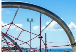
The steel arches are hot-dip galvanised inside and outside with lead free zinc. The galvanisation has excellent corrosion resistance in outside environments and requires low maintenance.
