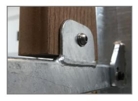
The WPC boards are attached to 70 x 45 x 3mm welded flanges with stainless steel M8 bolts, nuts and washers. These connections are not visible from the inside and create a strong and safe connection.
