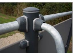
The connectors are made of die-cast aluminium.
