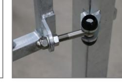
The hinges on the entrance gate are 16mm and made of Stainless Steel, the handle can be accessed from both inside and outside of the pitch but is constructed in such a way that it remains fully flat on the inside of the MUGA.
