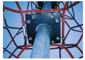
Corocord membranes consist of friction-proof rubberised material of conveyor belt quality with excellent UV resistance. Tested and compliant with REACH requirements for PAH. Embedded is a four-layered armouring made of woven polyester. The armouring and the two surface layers result in a total thickness of 7.5 mm.
