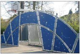
The goal measures ~140cm in depth and ~330cm in width with all posts made of galvanized steel with a hot dip galvanized surface treatment. The front frame is made with Ø48 tubing, and the backside of the goal uses 10 tubes with a diameter of ø38.
