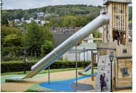
Curved and straight stainless-steel tunnel slides are supported by multiple steel rods to a center steel post. The tunnel slides are designed with perfect curve and inclination for a playful ride.
