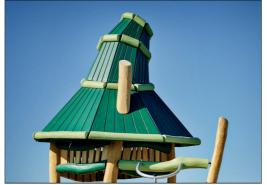
Transparent brown pigmented and colored parts, are coated with water-based paint and pigment that is environmentally friendly and with excellent UV resistance. The paint and pigment is in compliance with EN 71 Part 3.
