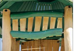
Max. fall height 197 cm Safety surfacing area 83.8 m<sup>2</sup> Total installation time 53.7 Excavation volume 4.53 m<sup>3</sup> Concrete volume 3.00 m<sup>3</sup> Footing depth (standard) 100 cm
