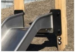
Slide interface panel of 19mm EcoCore™. EcoCore™ is a highly durable, eco-friendly material, which is not only recyclable after use, but is also made of +95% recycled postconsumer material from e.g., food packing waste in both core and colorful outer layer.
