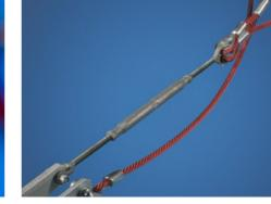
The spacenets' main bearing ropes are equipped with an additional safety feature: should the main connections fail, the safety rope prevents collapse of the structure.
