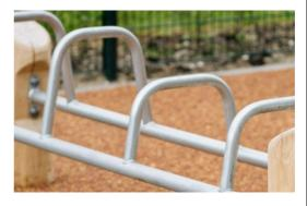
Bars intended as grips during exercises are made of hot-dip galvanised steel ø38mm. A great diameter to support the wrist when doing dips or handstands.
