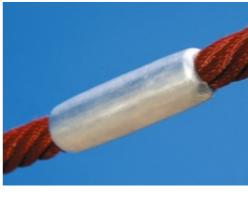
The aluminium swages of the net are double conical with rounded ends and are as small as safety allows. The overall net design aims at keeping metal parts within the net to an absolute minimum, both in size and number, to provide the best possible rope climbing experience.
