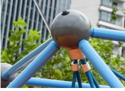
The metal parts are made from high-quality steel consisting of hot-dip galvanisation on both the inside and outside and also includes leadfree zinc and an additional layer of powder coating. This ensures both excellent corrosion resistance and colourful design expression. LUNA
