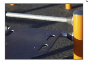
All decks are made of High Pressure Laminate HPL with a thickness 17.8mm and non skid surface texture according to EN 438-6. KOMPAN HPL has high wearing strength to ensure long lifetime in all climates.
