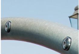
The steel structure are hot dip galvanized inside and outside with lead free zinc. The galvanization has excellent corrosion resistance in outside environments and requires low maintenance.
