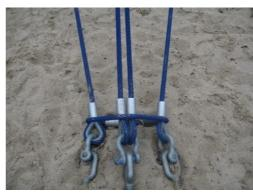
The huge spacenet structures are secured to the foundation with a system of three turnbuckles. Horizontal and vertical edge cables are fixed to individual turnbuckels, which then connect to individual steel anchors. This system ensures that each edge cable can be tensioned separately and increases structural safety by way of independent anchoring.
